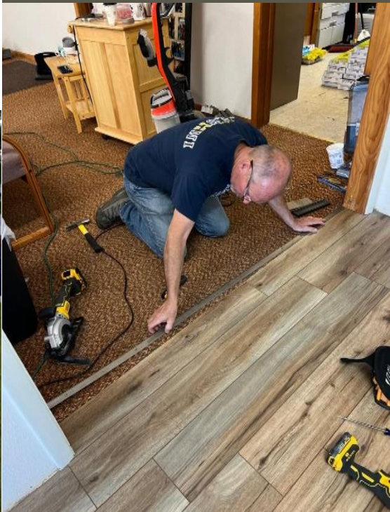
Photos Below: Installing flooring at a Hispanic Church in Grandview, WA
